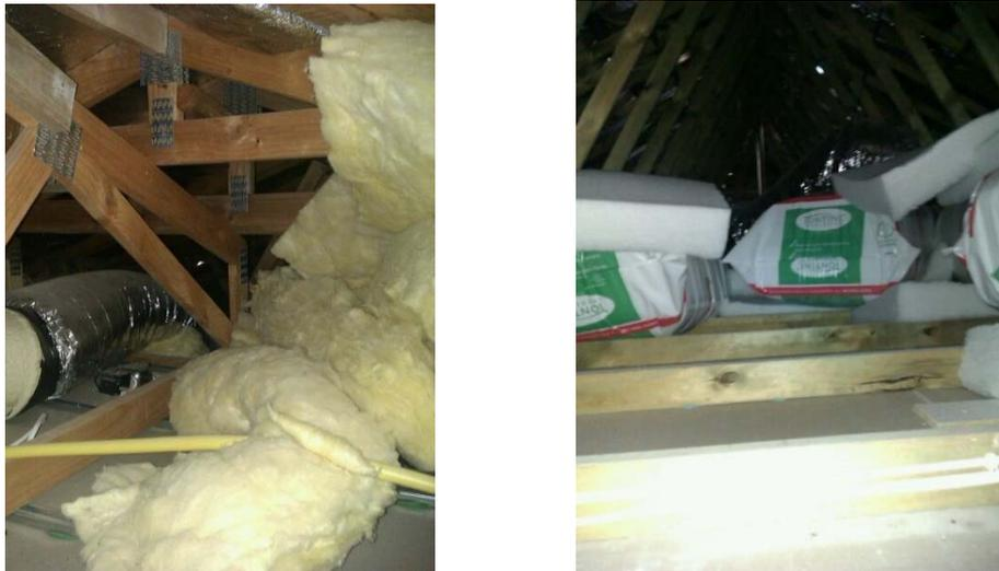
Fig. 3. Examples of ceiling insulation rated as poor.
