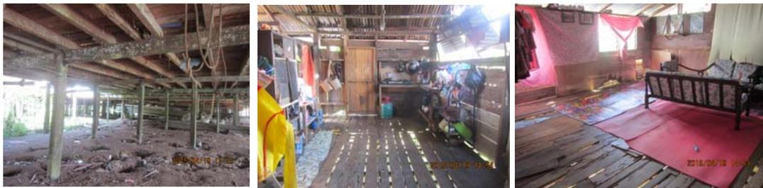
Fig. 6. High stilts of the Rasau longhouse, Serian. The longhouse does not depend much on mechanical ventilation where it was found that no mechanical ventilation or air conditioner were installed.
