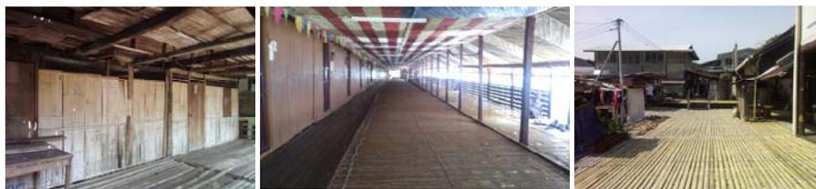
Fig. 8. (a) Split bamboo walls of the Benuk longhouse; (b) Split bamboo floor of the covered gallery in Mongkos longhouse; (c) Split bamboo floor of the open veranda in Annah Rais longhouse. All three longhouses are Bidayuh longhouses.
