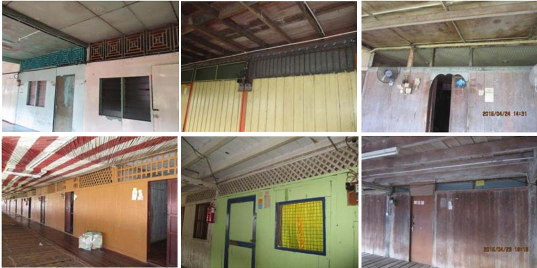
Fig. 3. Different styles of the fixed transom on top of the front apartment wall facing the long covered gallery in the longhouse.
