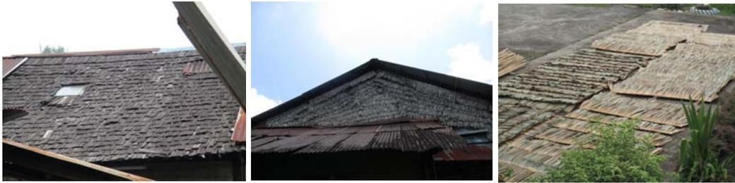
Fig. 9. (a) Timber shingles roof; (b) Wall coverings from sago palm thatch; (c) Sago palm thatch dried under the sun.
