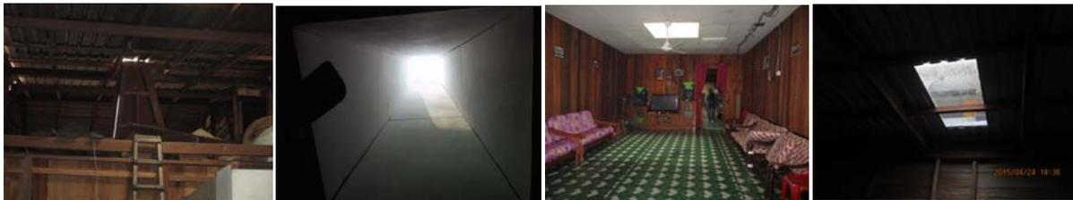
Fig. 10. (a) The roof light tunnel as seen from the side; (b) The interior of the roof light tunnel; (c) The roof light tunnel lights up the living room of one of the apartments in the Rumah Ah Soon longhouse; (d) Transparent roof coverings allow natural daylight to light up the dim longhouse.
