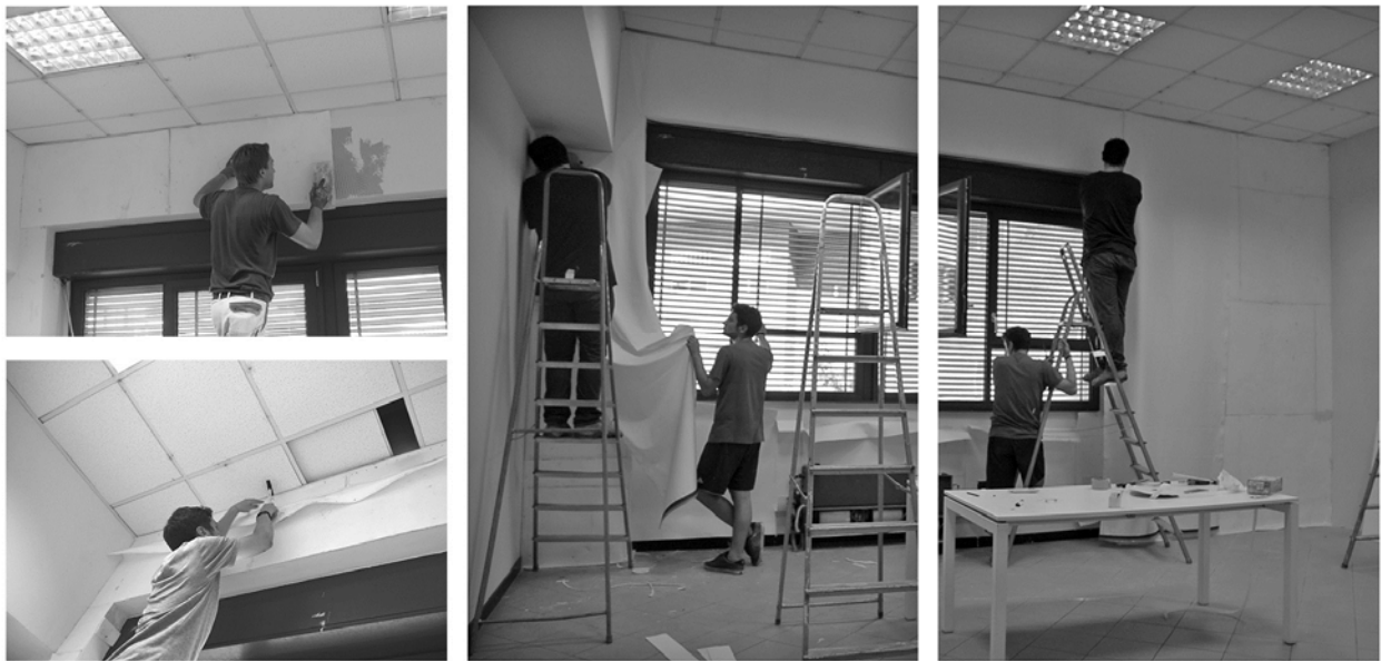
Fig. 4. Test of the insulating wallpaper with the final solution for the tensioning system, July 2015.
