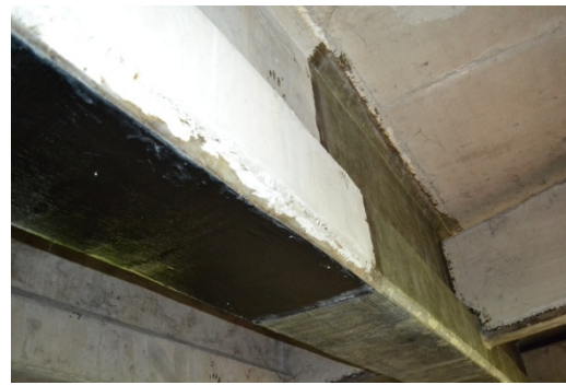
(b) Strengthened Girder using GFRP Sheet
