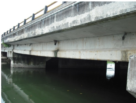
(a) Concrete Girder Bridge
