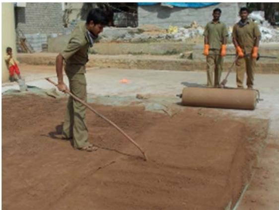
Fig. 4. Preparation of MSW by rolling to break lumps
