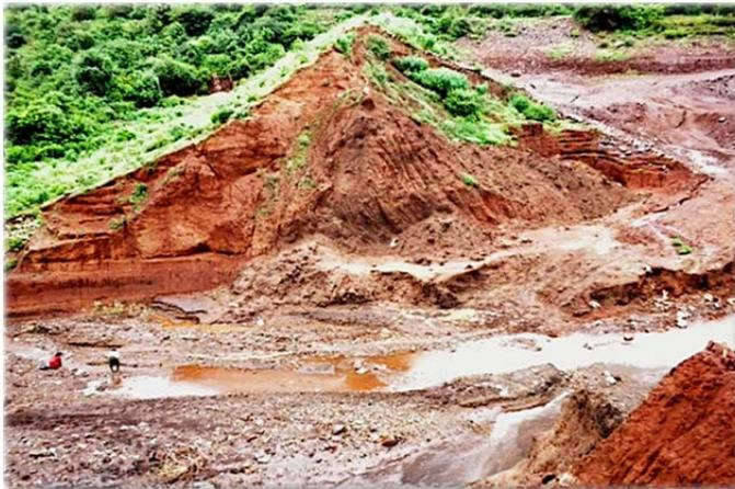
Fig. 1. View of breached portion of Ankamanahal dam during August 2011
