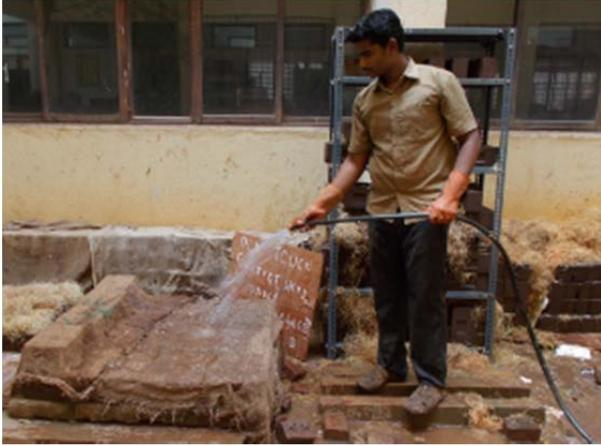
Fig. 8 View showing curing of blocks
