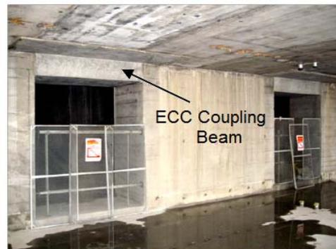
Fig. 5. ECC coupling beams for a 60-story reinforced concrete building – Osaka (Japan) [24]
