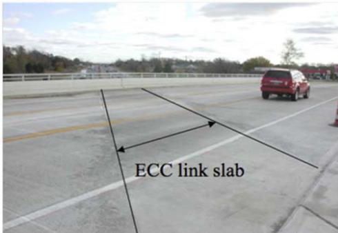
Fig. 4. ECC link slab in bridge deck replaces conventional expansion joints – Michigan (USA) [23]
